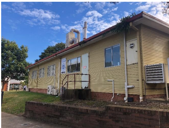
Figure 41. 1990s addition to the south of the original hospital building featuring weatherboard cladding, aluminium sliding windows and external stair.
