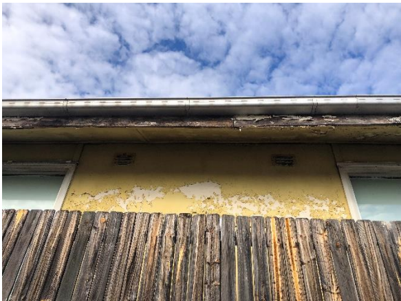
Figure 37. Close up of the northern elevation featuring peeling paint and deteriorated fascia boards.
